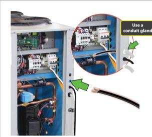
Connect Controller Unit Wiring (cont)
