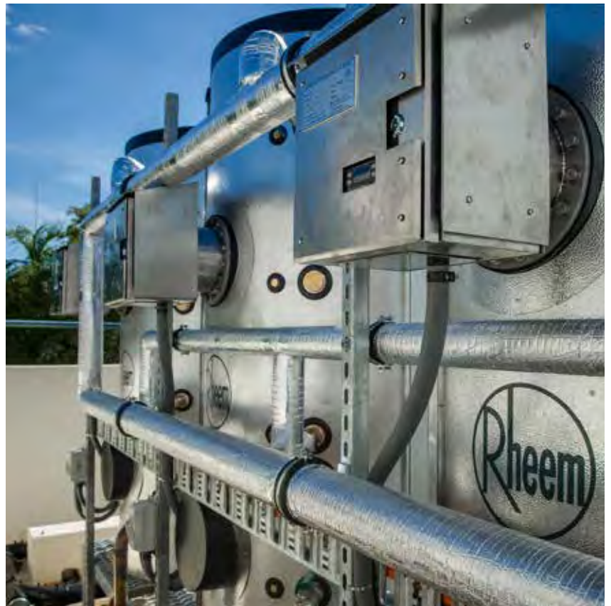
Rheem HS Series solar with electric boosting in the top of solar tanks. Katherine Hospital NT.
