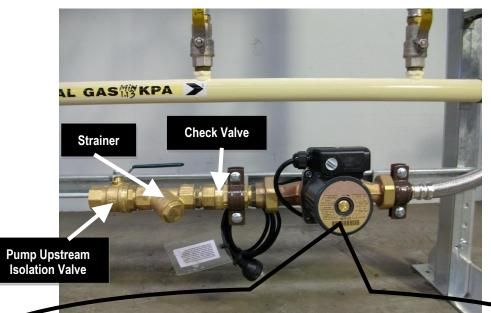
Basic Instruction for inline wet rotor Circulating Pump; Motor shall be "Horizontal"; Never Operate "Dry"; Loop cable down on exiting terminal box as shown; "Bleed" Pump; Confirm "Rotation"; "Free" shaft assembly, if necessary; Power Supply Timer is required to turn off pump automatically at least four (4) times daily for short periods; Clean Pump Suction Strainer regularly.
