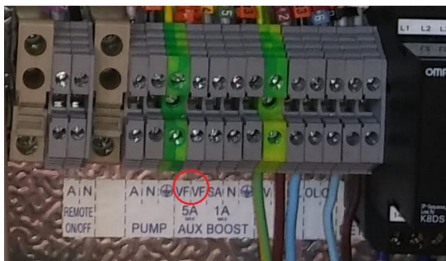
Picture of heat pump terminal strip
